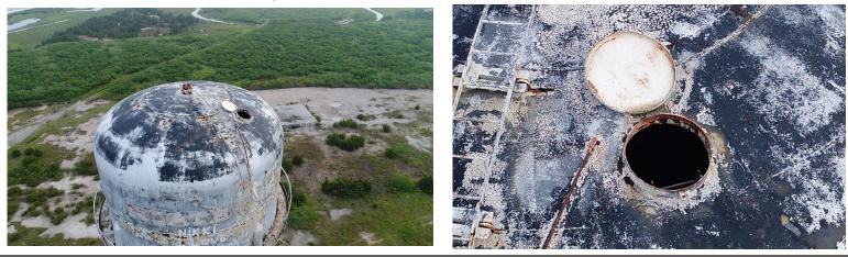
A UAV inspection is safer alternative than a multi-person crew and more cost effective way to inspect exterior tank conditions, coating, hardware and hatch integrity. This is also a great way to confirm and document a whole systems security and vulnerability potential.
