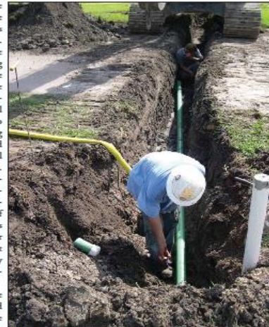
Vacuum sewer service lateral installation is simplified because lines are shallow and can easily be diverted over or under buried obstructions.
