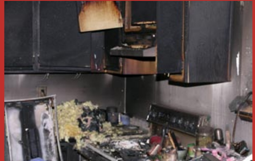
KITCHEN FIRE WITHOUT SPRINKLERS
