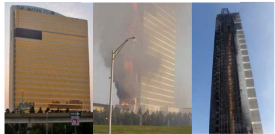
Atlantic City (US) – 2007 Hot-work sparks from roof in cavity wall ACM cladding, PS insulation
