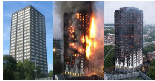
Grenfell (UK) – 2017 Source: Interior
