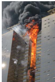
Korea 2010 Electrical fire
