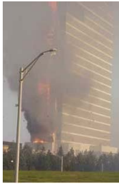
Atlantic City (US) – 2007 Hot-work sparks in cavity wall
