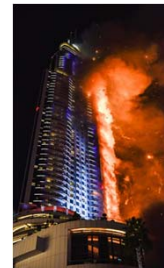
Dubai 2015 Electrical short-circuit
